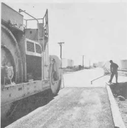
UNDER MANY tons of pressure, the gravel is rolled forming a compact surface. BAO HOPI tonelada di presion, e graniet ta worde lorá formando un capa duro.
